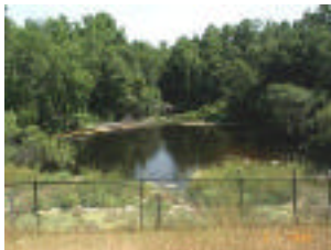
This overflow reservoir lies north of Lake Grady and flows into Bell Creek. USF
